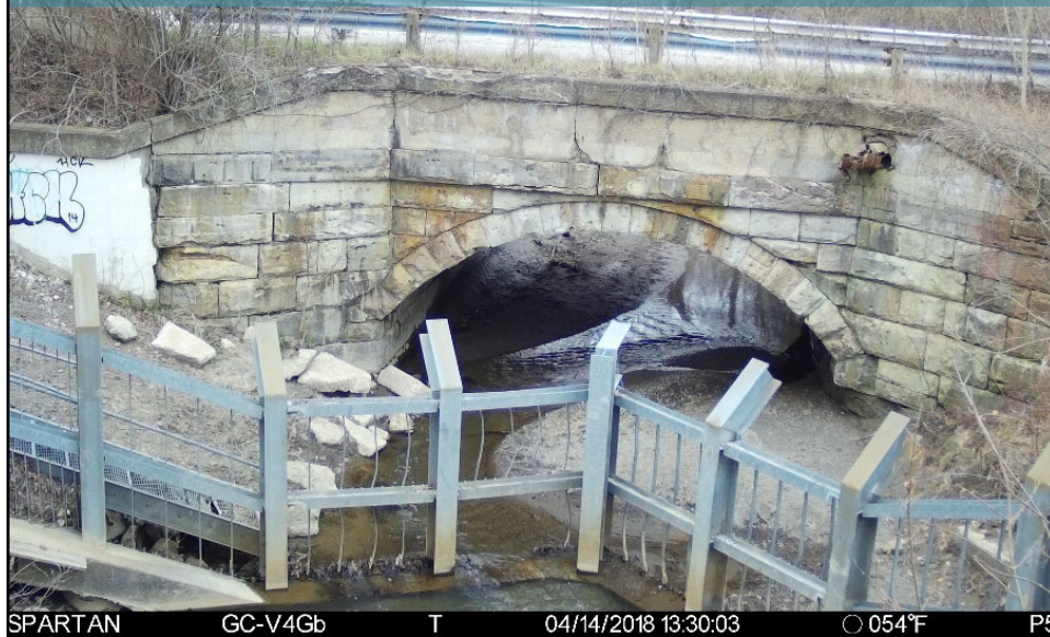
April 14, 2018: Debris Rack is Clear Before the Storm Event
